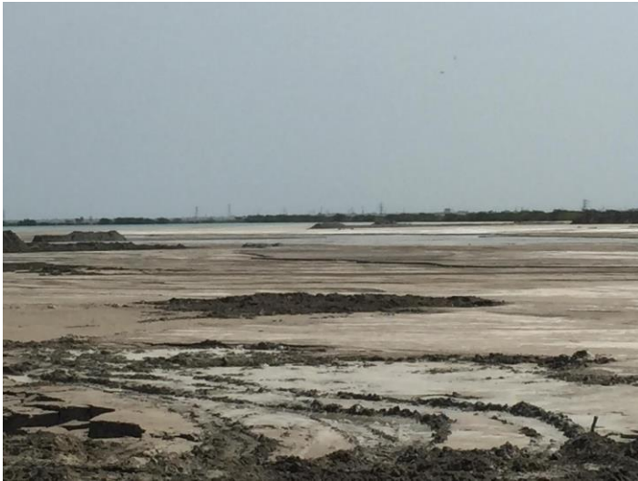
(a) North Chennai Thermal Power Station Ash Pond
